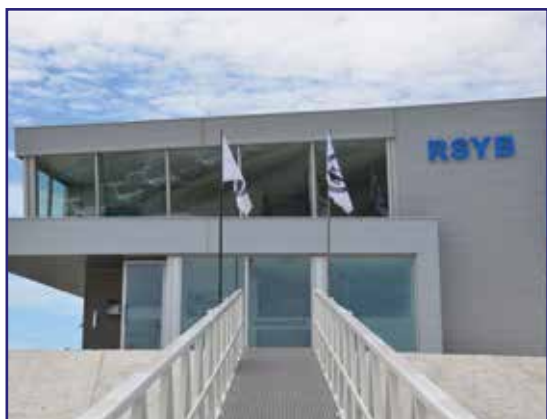
Havenkantoor Capitainerie Harbour masters office
